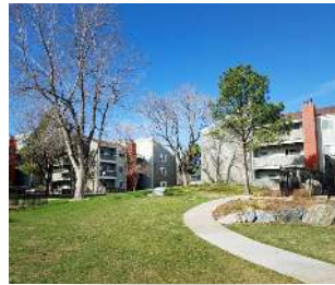
GROVE AT CITY CENTER 420 UNITS
