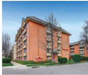
BRITTANY HOUSE 68 UNITS
