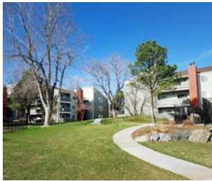
GROVE AT CITY CENTER 420 UNITS
