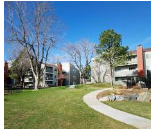
GROVE AT CITY CENTER 420 UNITS
